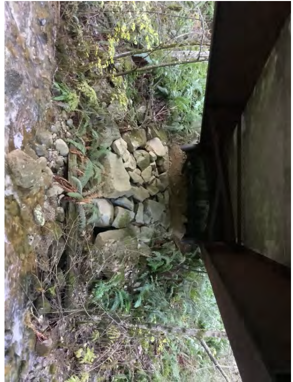
Right Bank Abutment when facing downstream
